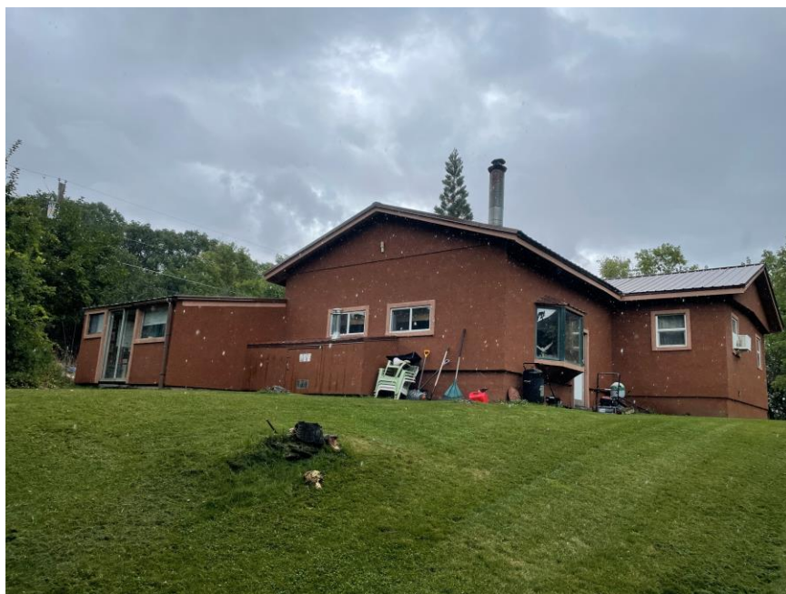
Exterior, facing southeast.
