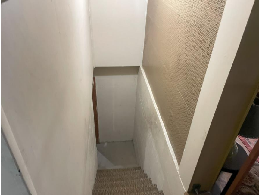
Stairs down to basement.
