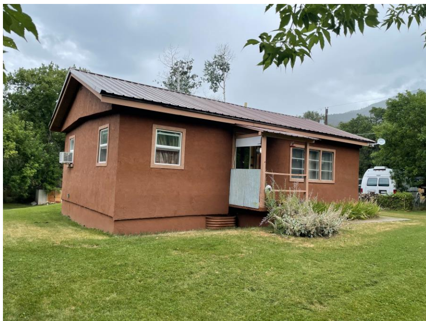
Exterior, facing northeast.
