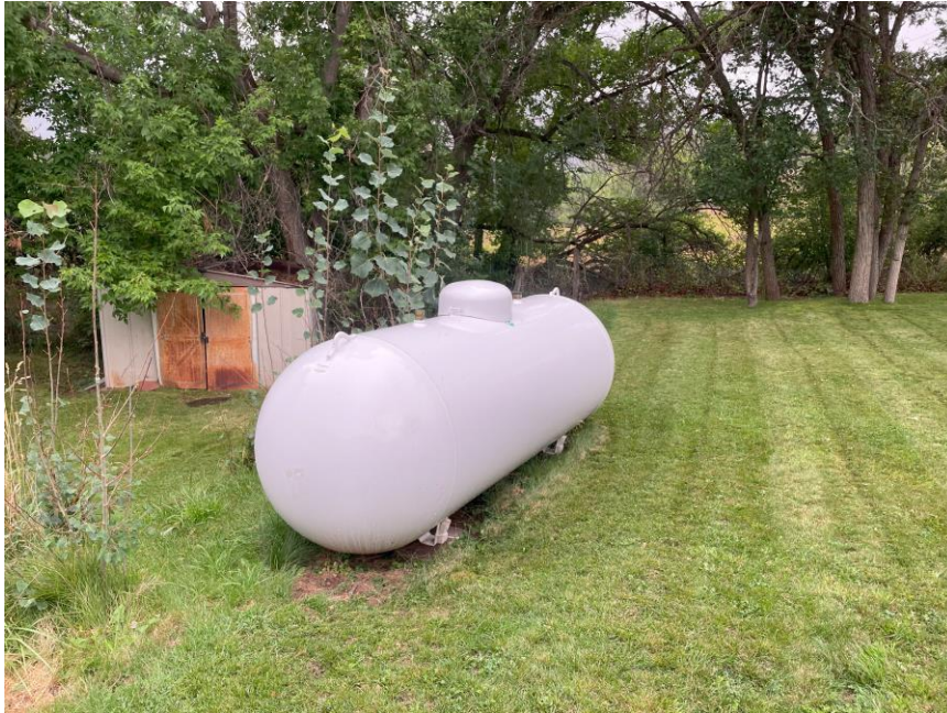
Propane tank and poor condition shed.
