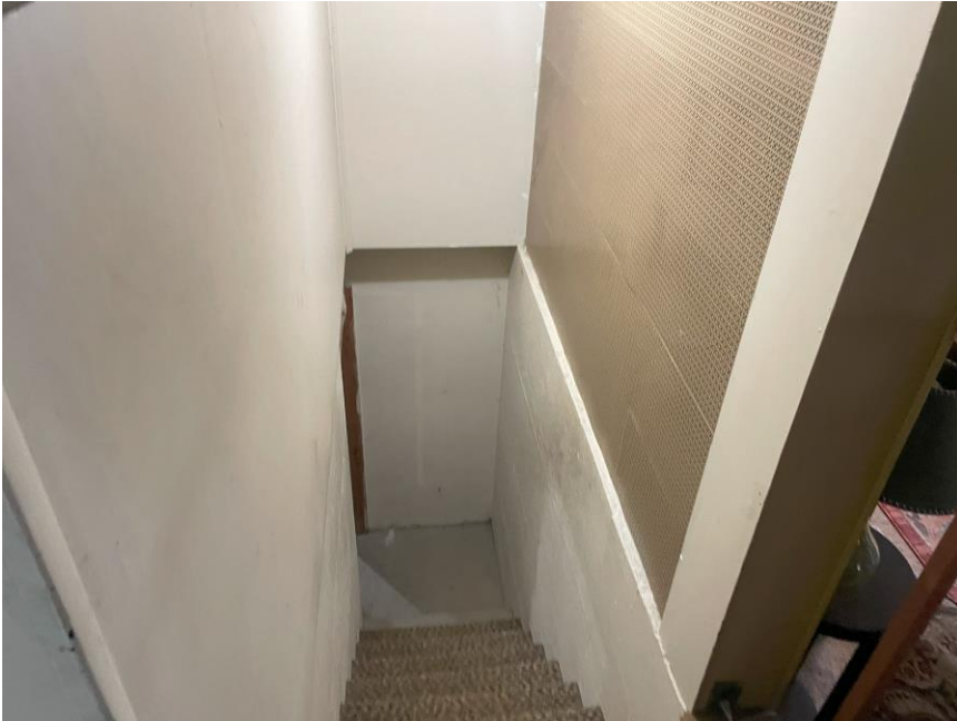
Stairs down to basement.
