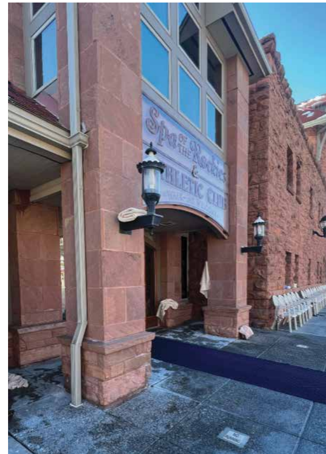
④ Athletic Club Pool Entrance ID Wall Sign - Photo - Scale: NTS
