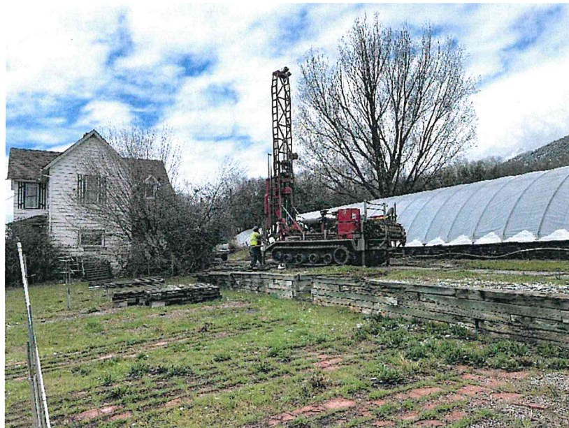
Drill rig at TH-4 looking northwest
