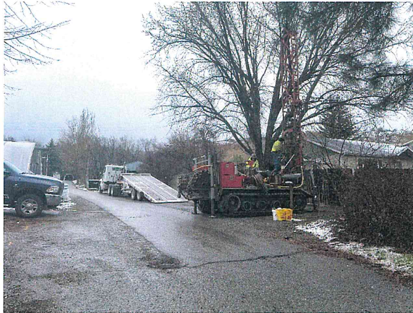
Drill rig at TH-6 looking north
