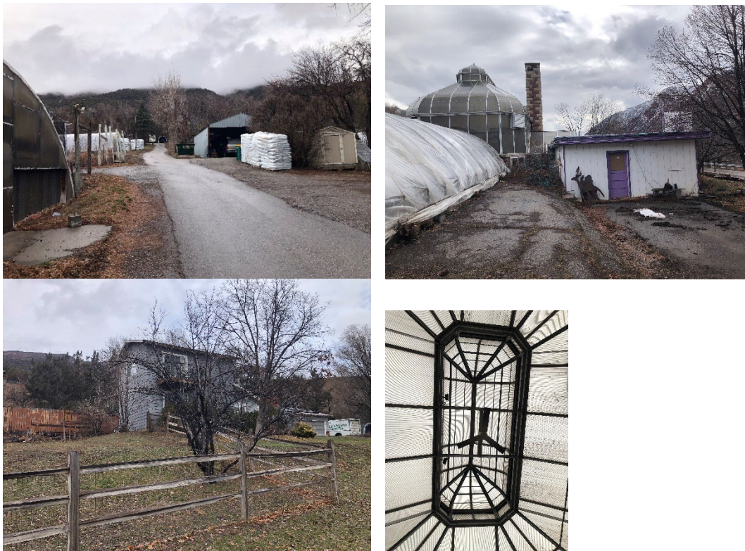
Top-left, moving clockwise: The view toward the north from near the entrance; the historic greenhouse, newer hoophouses, and accessory structures; one of the inhabited single-family homes on the property; upward view inside the historic greenhouse.
