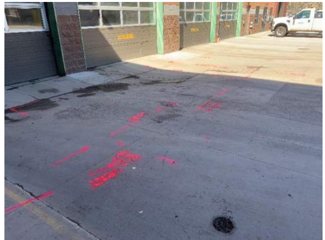
Site photo showing vent lines traced from nearby above ground vent. Lines were unable to be traced all the way to tanks and could not be seen using GPR.
