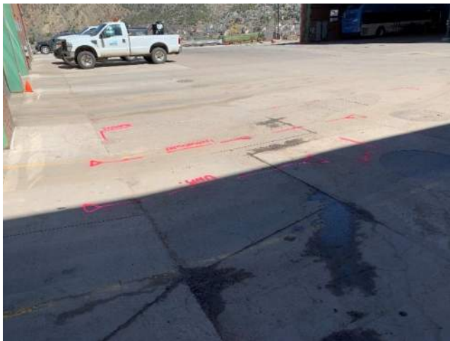
Site photo showing two unknown lines at north ends of tanks. Lines were found using passive sweeps and depths were unable to be verified. Lines did not extend past approximate centers of tanks and are believed to be associated with tanks.
