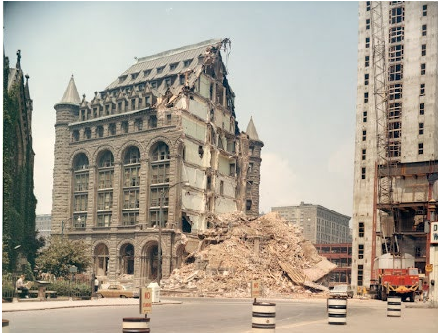
Demolition Erie County Savings Bank, Buffalo, NY, 1968 Packet Page 8
