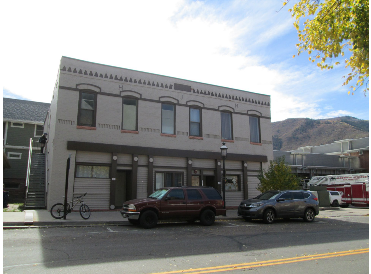
412 8 th Street, HJH Building, landmarked on September 17, 2015.
