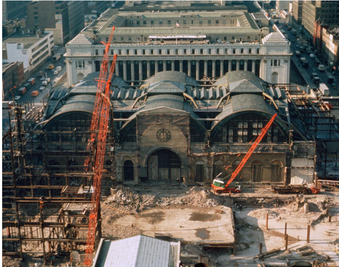
Demolition of Historic Penn Station, New York City, NY, 1963-1966
