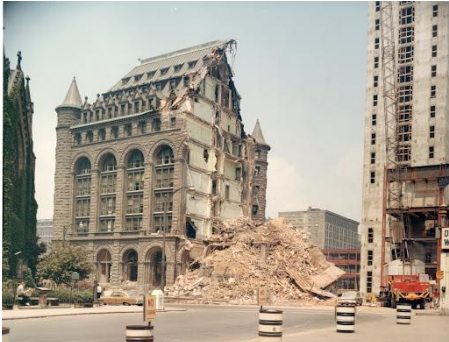
Demolition Erie County Savings Bank, Buffalo, NY, 1968 Packet Page 39
