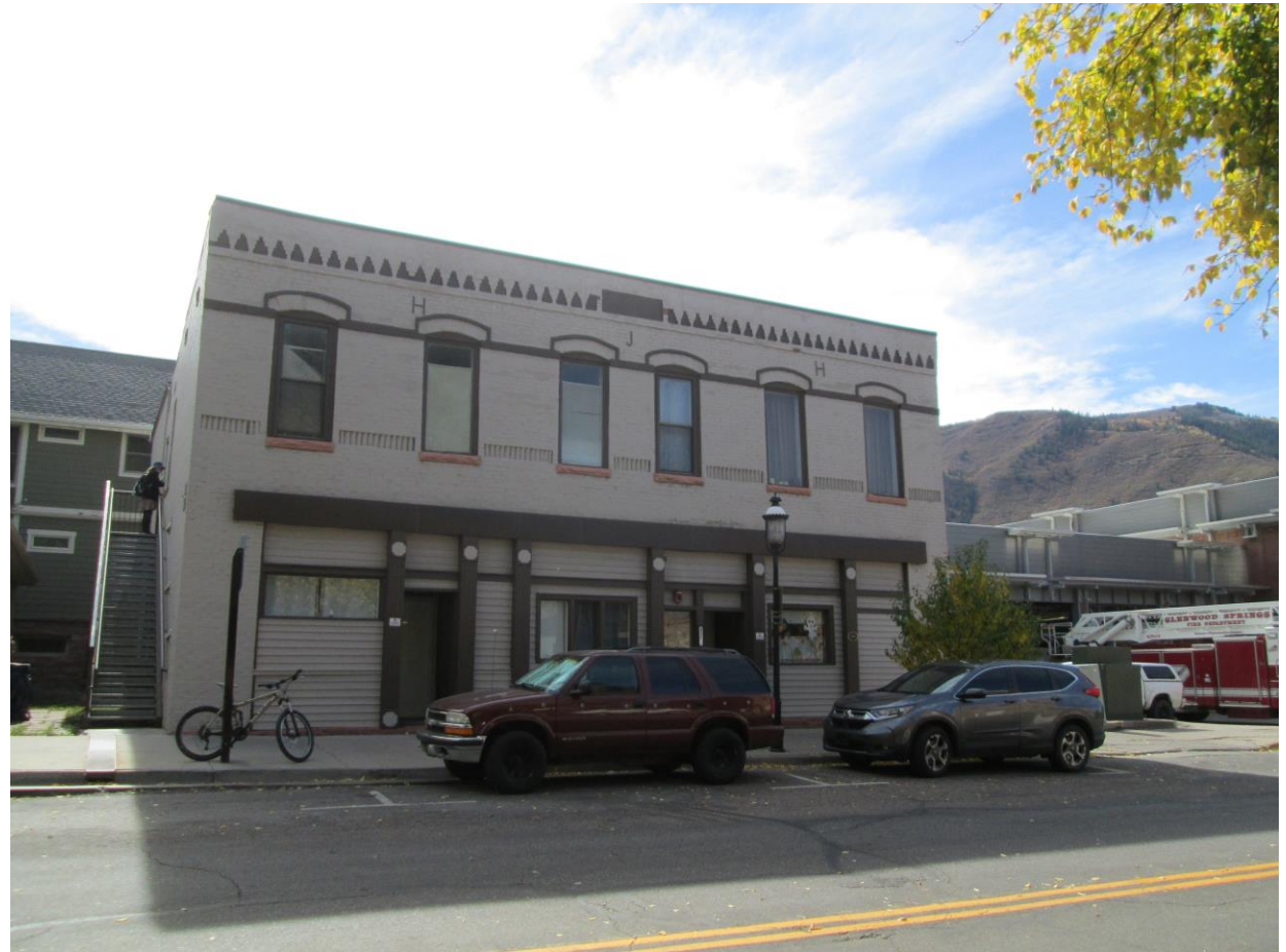
412 8 th Street, HJH Building, landmarked on September 17, 2015.
