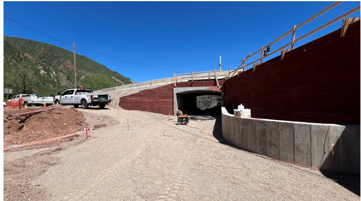
27th Street pedestrian tunnel portal, Northside (Left) Southside (Right)
