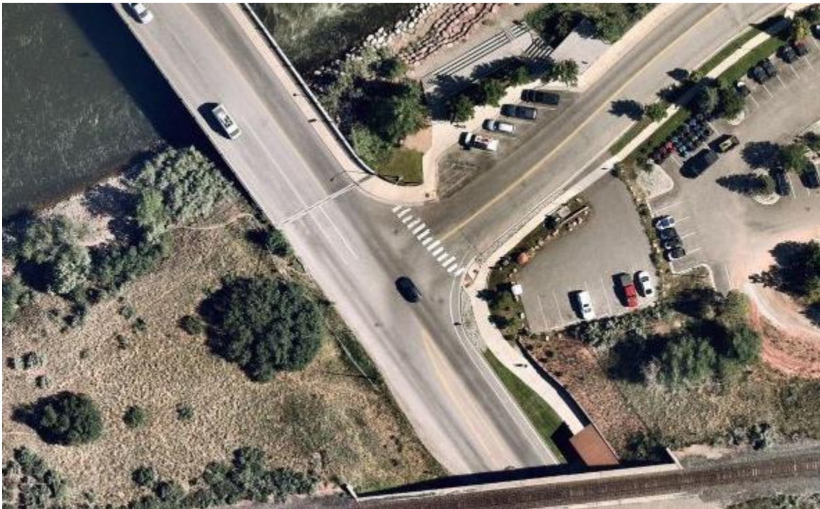
Devereux Road and Midland Avenue (#3)
