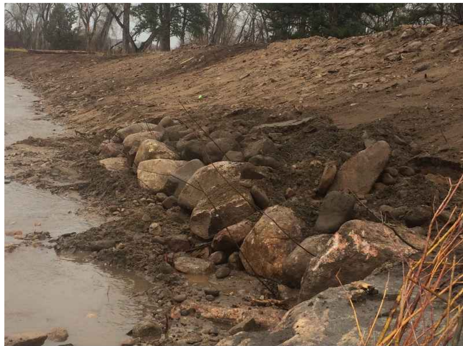
WILLOW CUTTINGS IN BANK STABILIZATION
