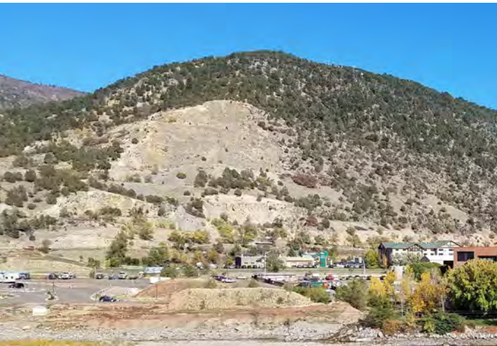
Holly Quarry Site
