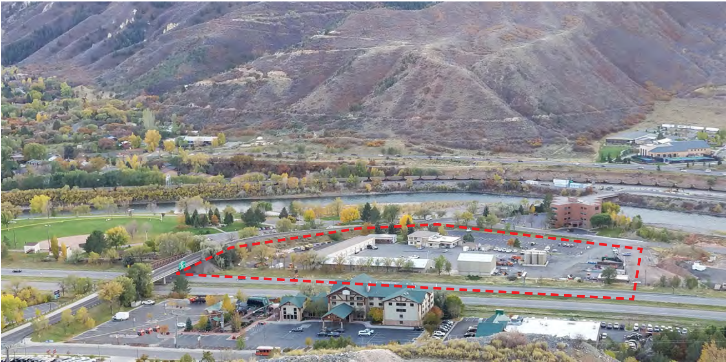
The CDOT Engineering & Maintenance Center
