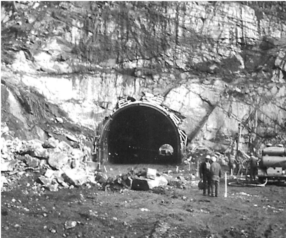
Construction of Glenwood Canyon Railroad
