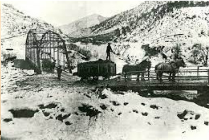
South Canyon Bridge, 1923
