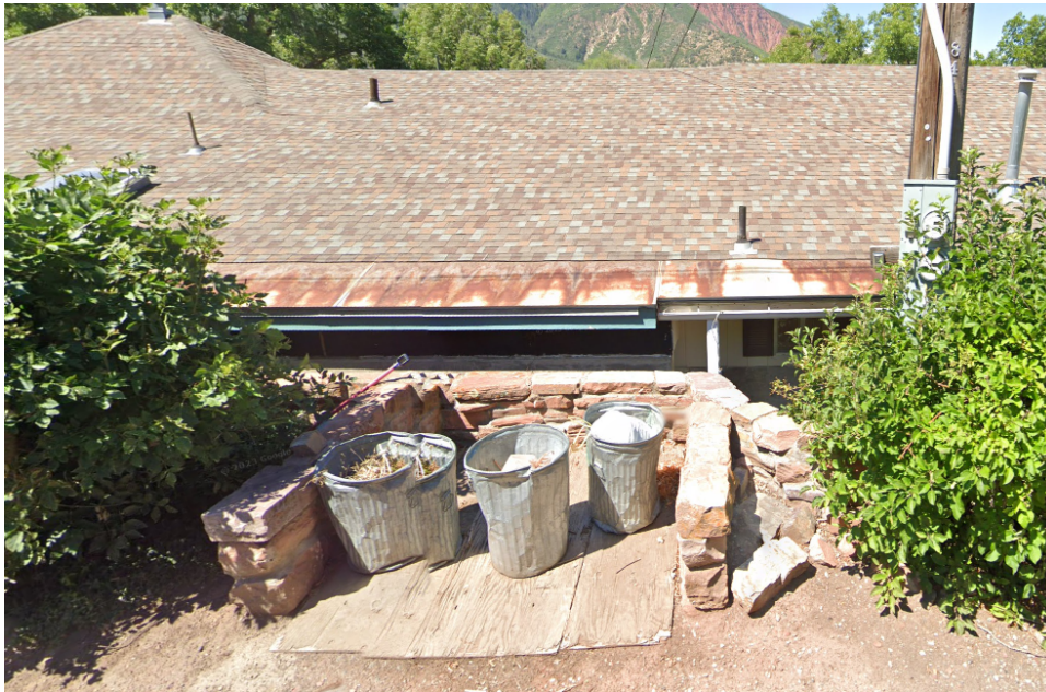
Above: Looking W – 707 9 th Street on Minter, north of previous picture at center of property line.
