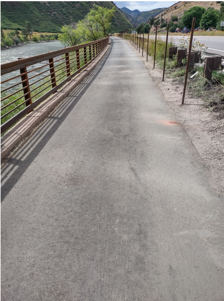
LoVa Trail “Meet Me In The Middle” Nearing completion, fall 2023 Looking west
