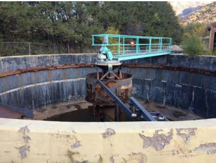
Former Waste Water Treatment Plant
