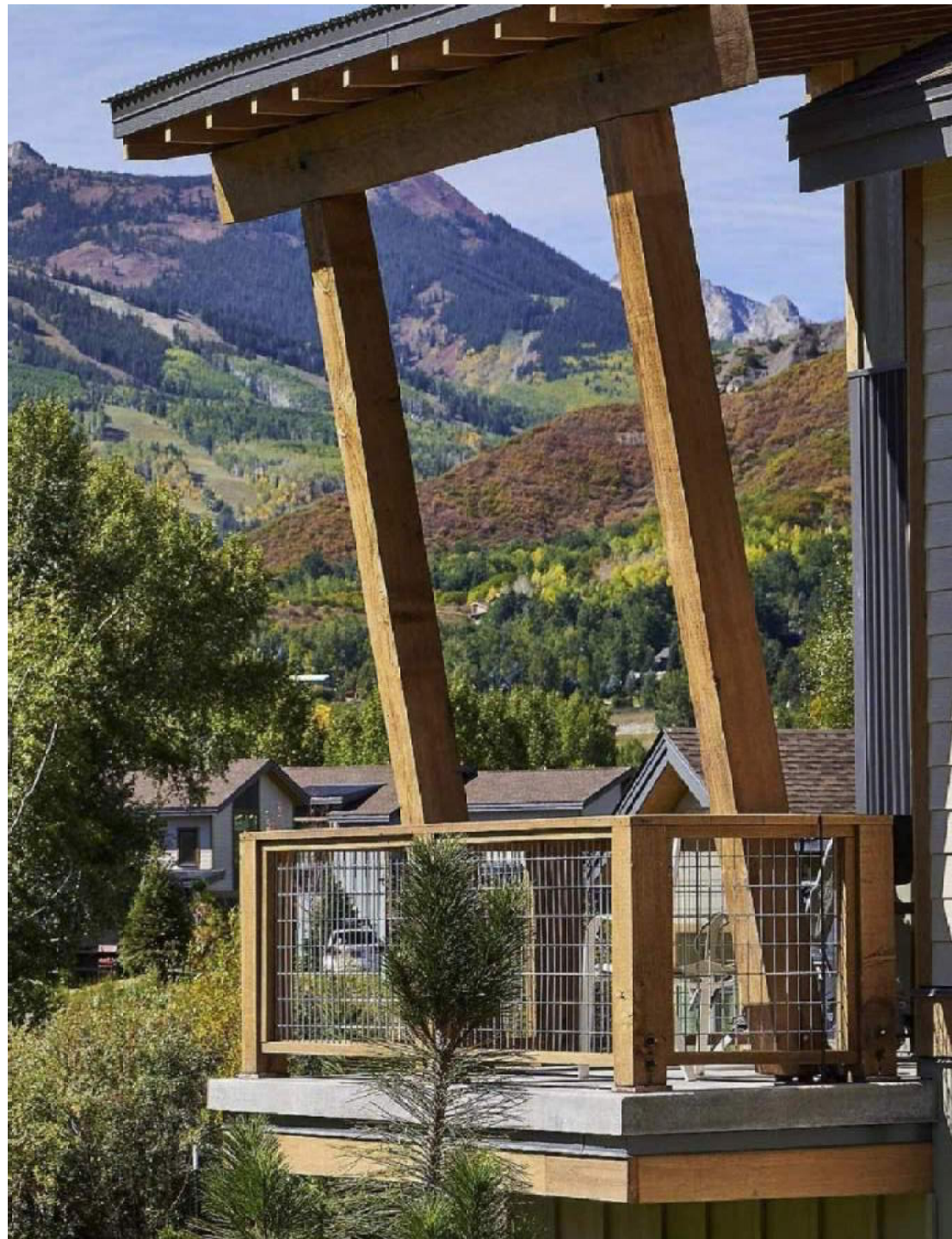
TIMBER STAIRS AND RAILINGS w/ GALVANIZED STEEL MESH INFILL
