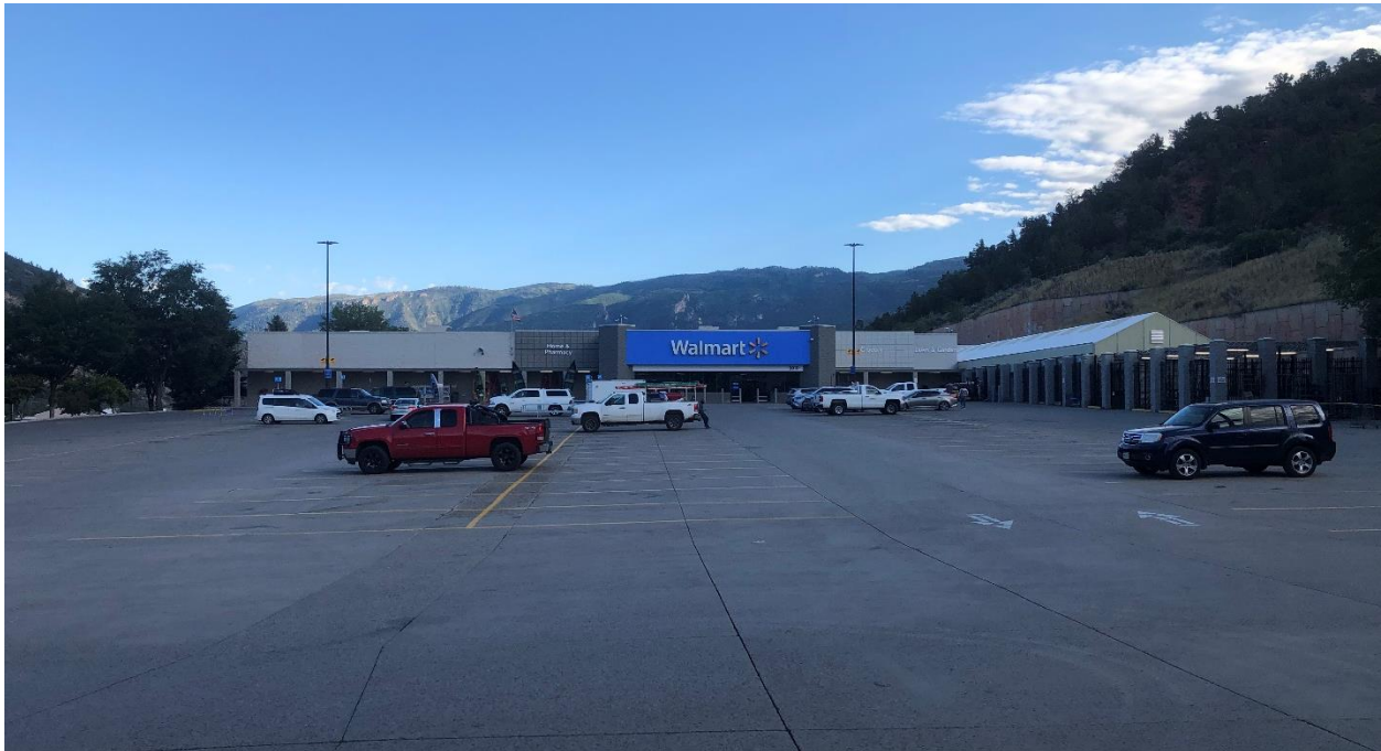
Existing signage looking north (the south elevation of the building)
