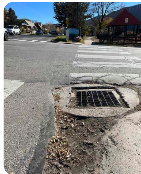
Existing drainage inlets on Blake Avenue.
