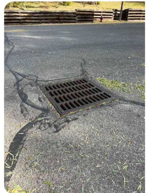
Existing storm sewer is located throughout the project limits
