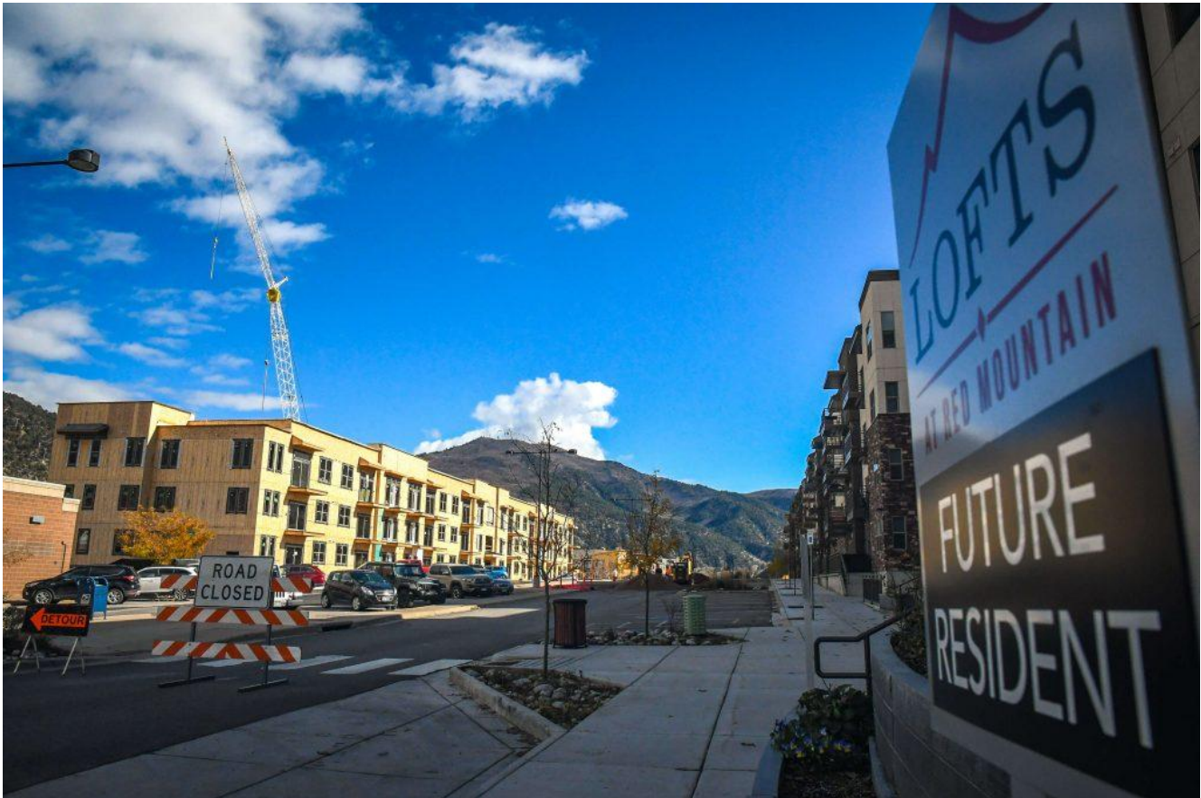
Construction crews continue work at The Lofts apartments in the Meadows shopping center in 2021 Chelsea Self/Post Independent
