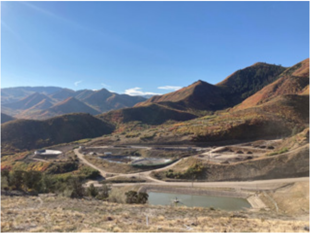
Landfill in South Canyon
