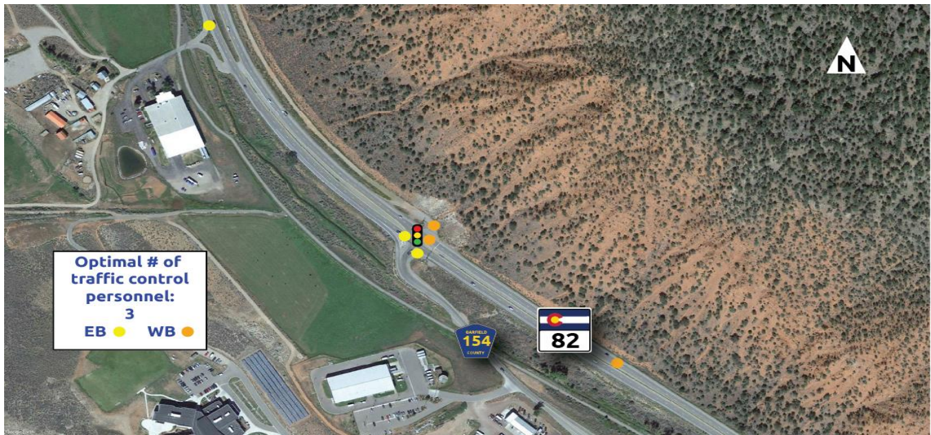
Figure 2.21 SH 82 Closure Point at CR 154
