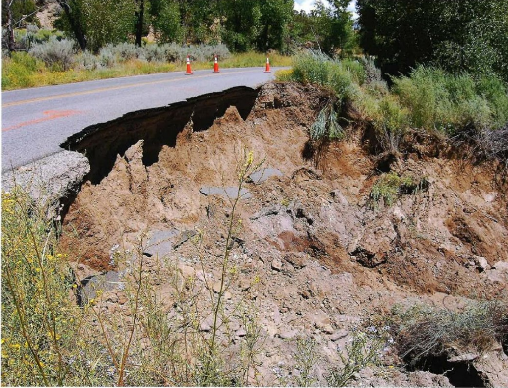
Erosion on County Road 237 near Harvey Gap in 2016
