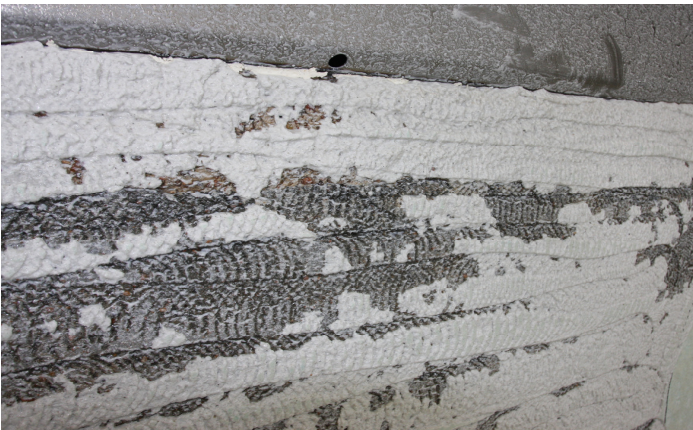
Pool Surface After Hydro-Blasting
