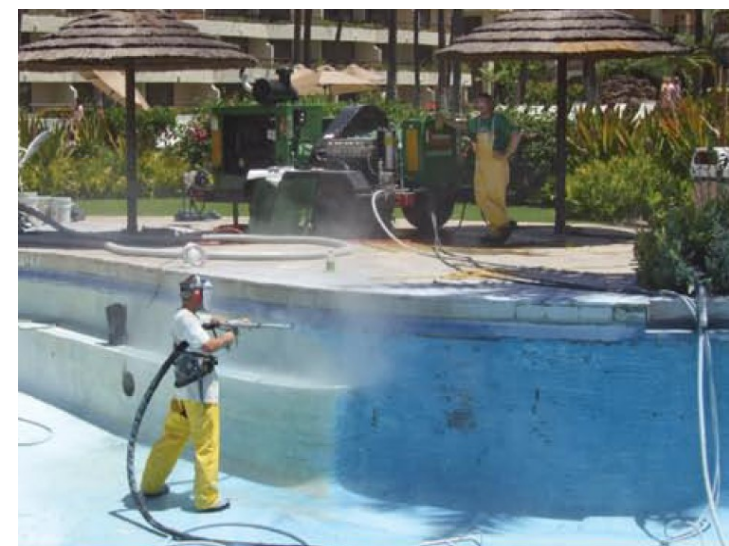
Hydro-Blasting removing pool paint
