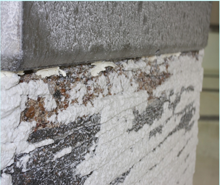
Removal of soft and deteriorated plaster at Prairie Band Potawatomie Indian Nation, KS
