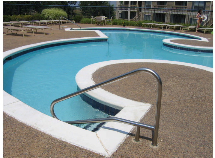
Pool re-plastered by Mid-America Pool Renovation, Inc.
