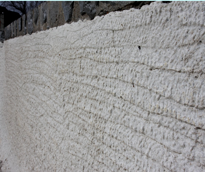
Residential Plaster Prep Overland Park, KS
