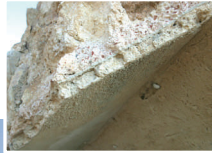
Plaster aqueduct interior
