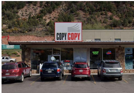
Roof sign (attached)
