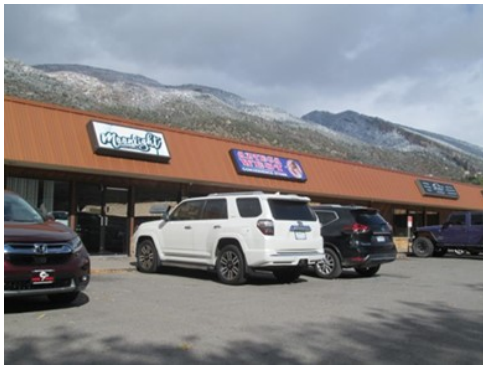
Wall sign (attached)
