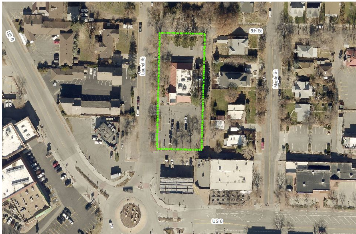
Photo of property location
