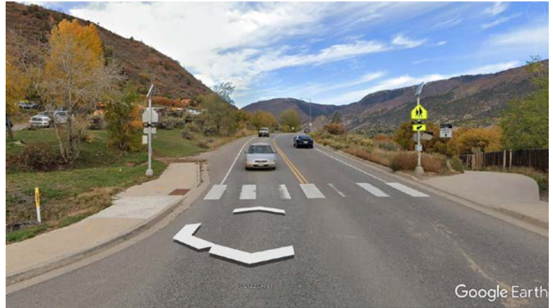
Figure 3: RRFB Installation on Midland Avenue near 13 th Street.
