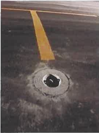
Tie Down Anchor Example
