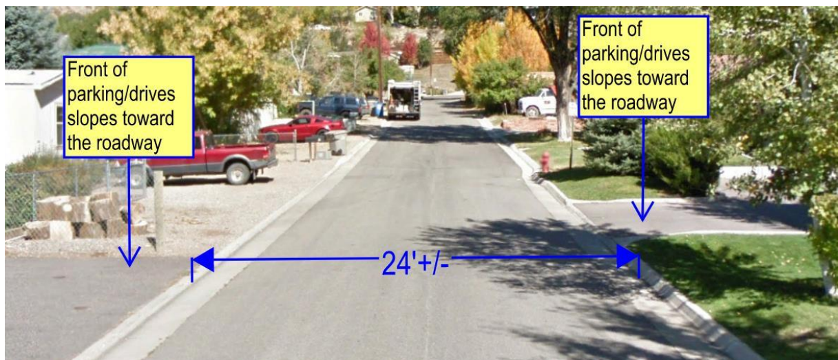
Figure 2: CR#135 Street Section
