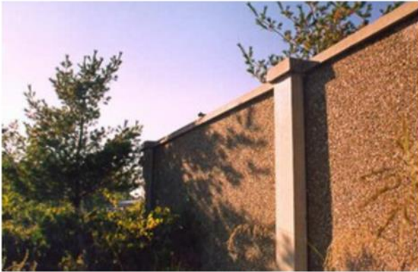
Figure 140. Noise wall horizontal cap
