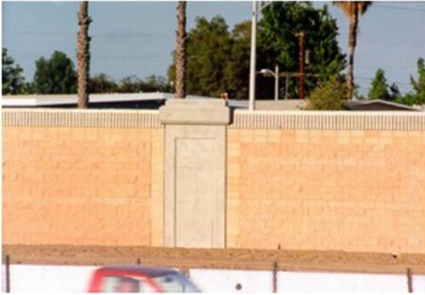
Figure 139. Noise wall horizontal cap
