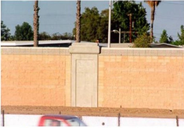
Figure 139. Noise wall horizontal cap
