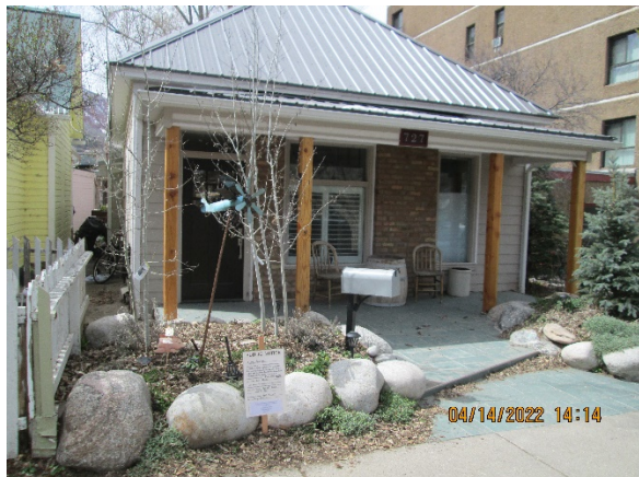
Photo of primary structure, from Blake Avenue
