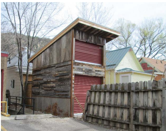
Finished shed, photo from alley
