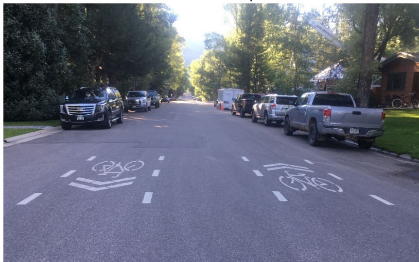
FIGURE 2: "SUPER SHARROW" PAVEMENT MARKING IN ASPEN, CO INDICATES PRIORITY & POSITIONING FOR BICYCLISTS ON SHARED ROADWAY.
