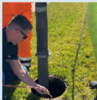
Vacuum removal of debris
