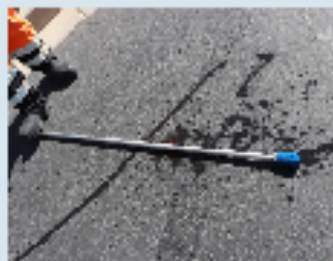
Wand used to loosen debris
