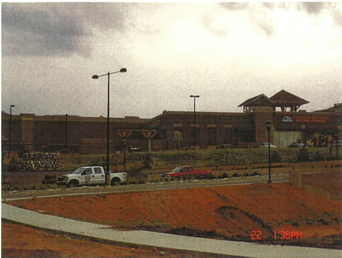
Photograph #: 1 Date: May 22, 2006 Direction: Facing east southeast Subject: View of the Site.
