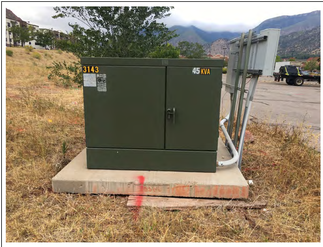
Photograph 9: View of pad-mounted transformer along the eastern Site boundary.
