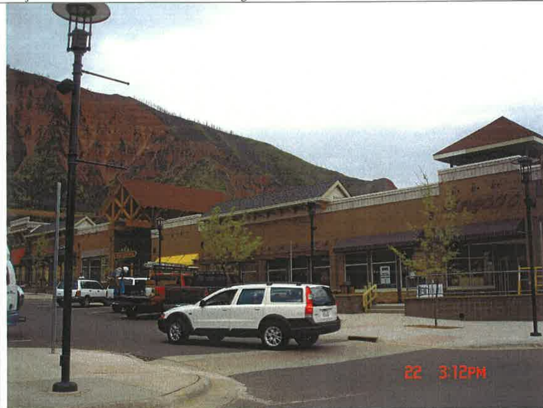
Photograph #: 6 Date: May 22, 2006 Direction: Facing southwest Subject: View of the multi-tenant buildings.
