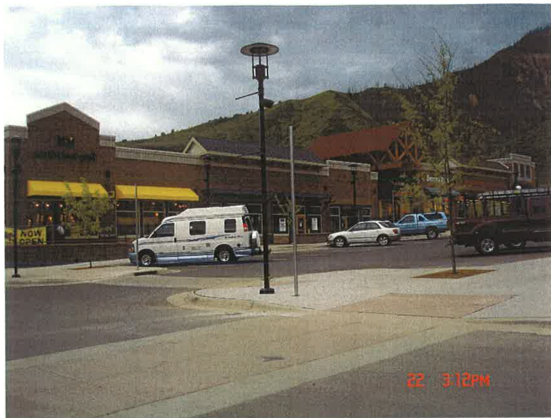
Photograph #: 5 Date: May 22, 2006 Direction: Facing southeast Subject: View of the multi-tenant buildings.
