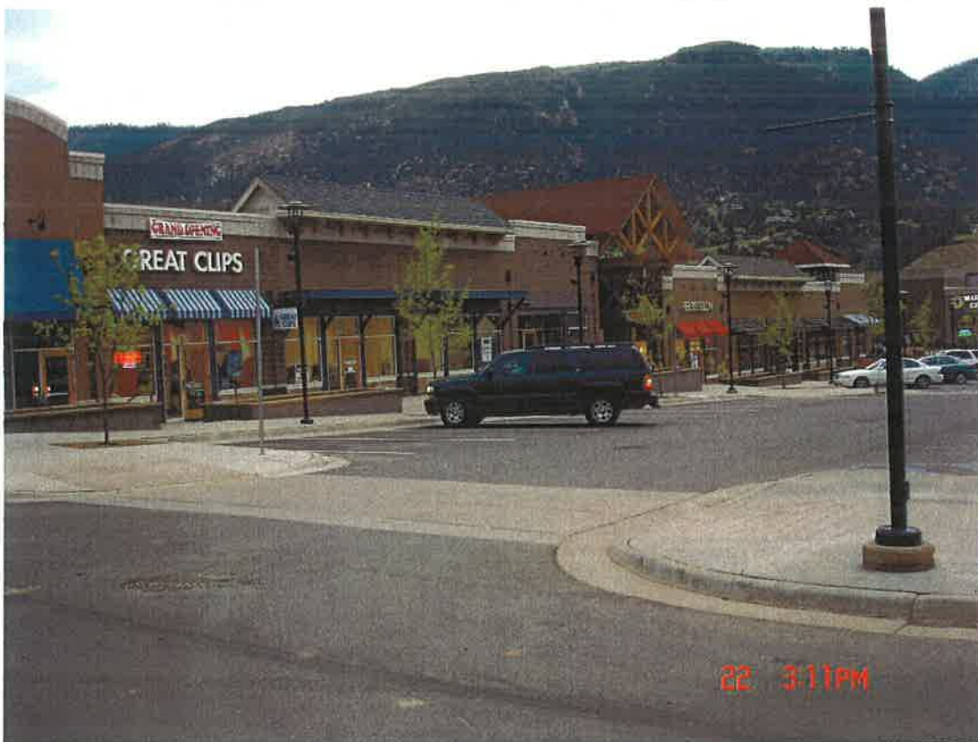
Photograph #: 4 Date: May 22, 2006 Direction: Facing northwest Subject: View of the multi-tenant buildings.
