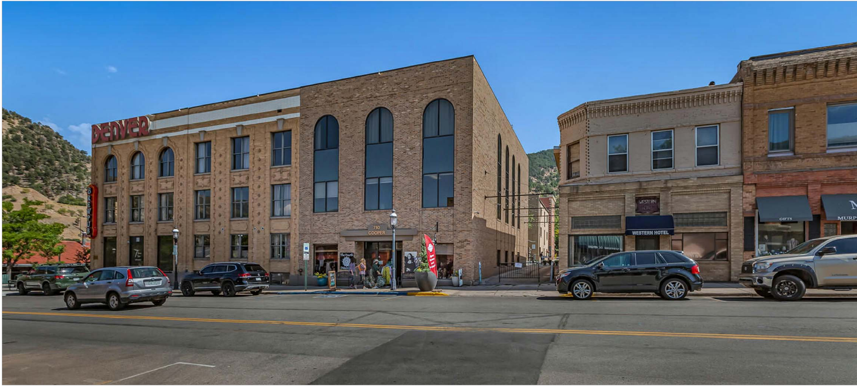
1 A0.2 NTS EXISTING IMAGE: COOPER AVENUE
