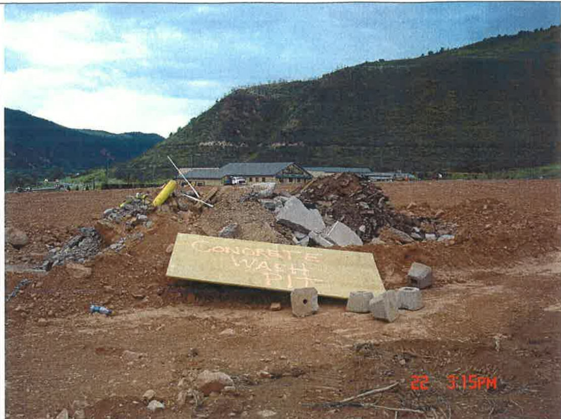
Photograph #: 7 Date: May 22, 2006 Direction: Facing east Subject: View of the remaining construction debris.
