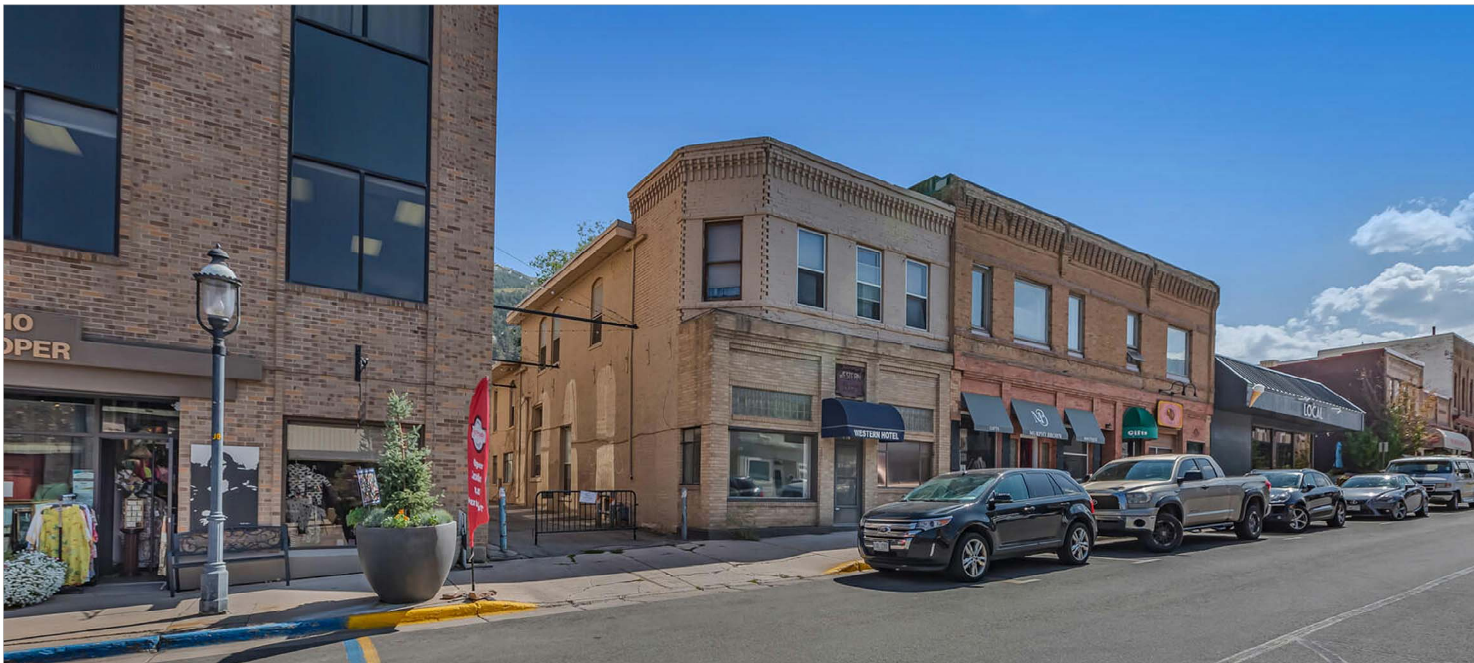
3 A0.2 NTS EXISTING IMAGE: COOPER AVENUE
