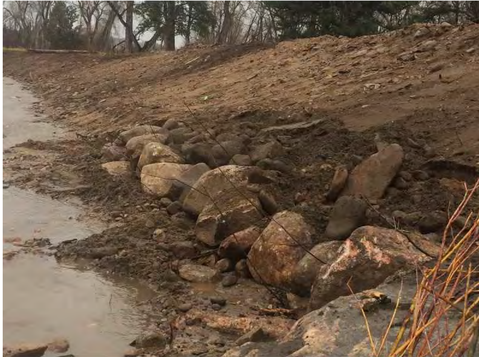
WILLOW CUTTING IN COBBLE TOE EXAMPLE
