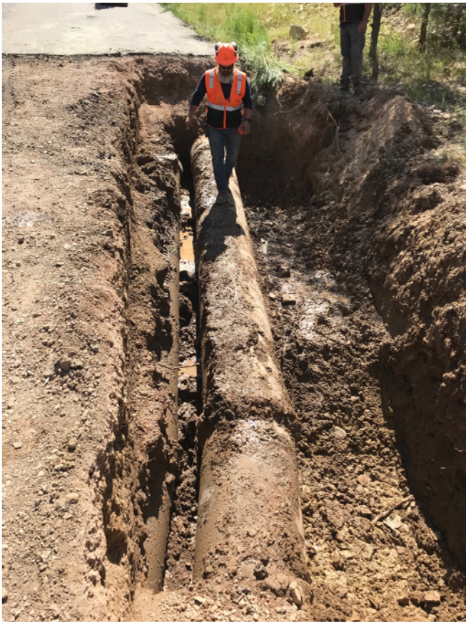
Raw Water Line Break 2020
