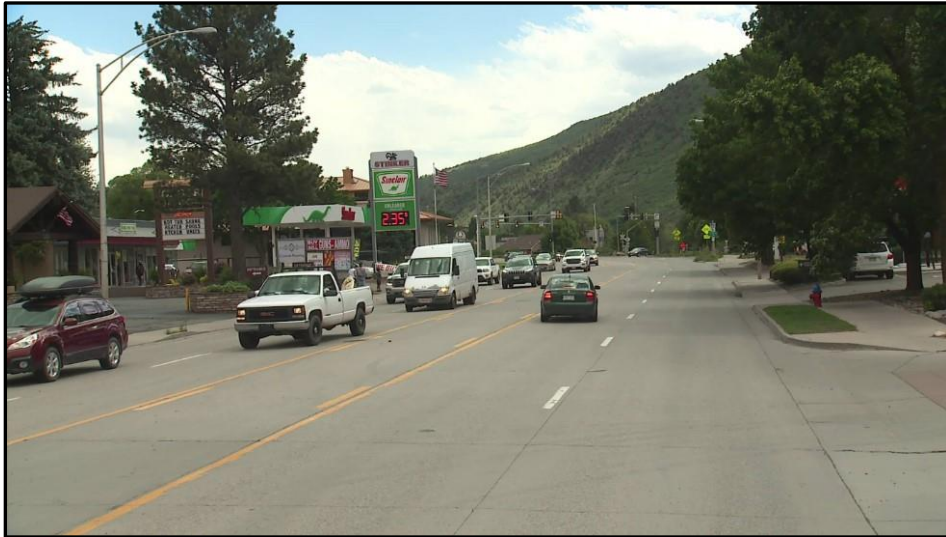
Image 2 – Looking South from 150' North of the Project Access
