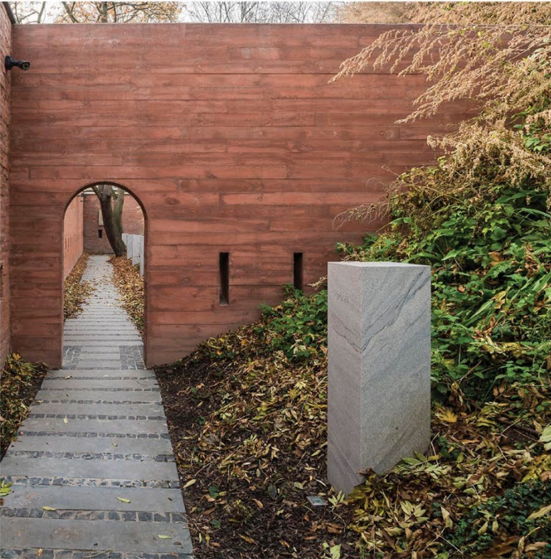
Stained Boardform Concrete
