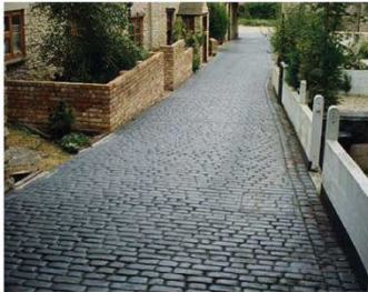
Stamped Concrete Matte Finish (dark integral color concrete)
