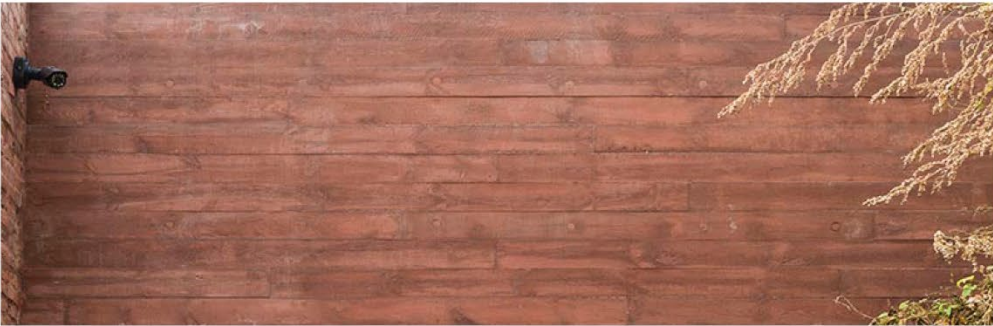
Stained Boardform Concrete
