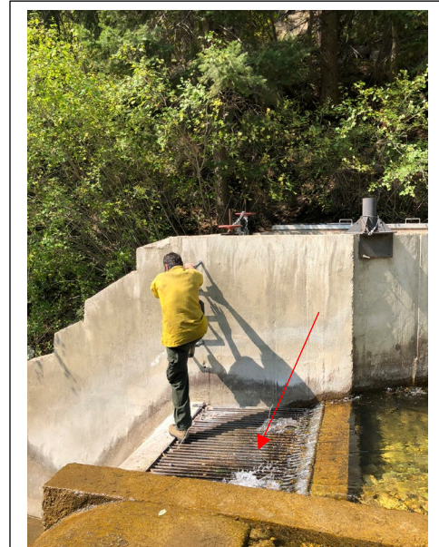
Replace bolted-on Grizzly Screen with plate.
