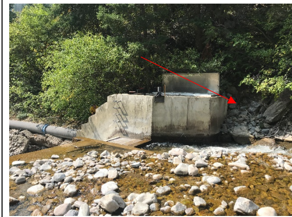
Concrete loose slopes to prevent sidcutting behind diversion.
