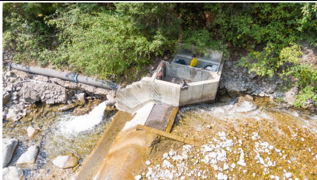
UAV photo of Diversion
