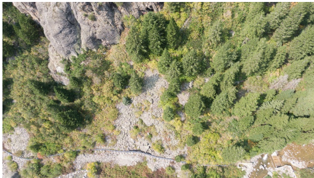
UAV photo of pipeline
