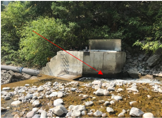
Cobble and debris removed in front of Coarse Debris Screen.
