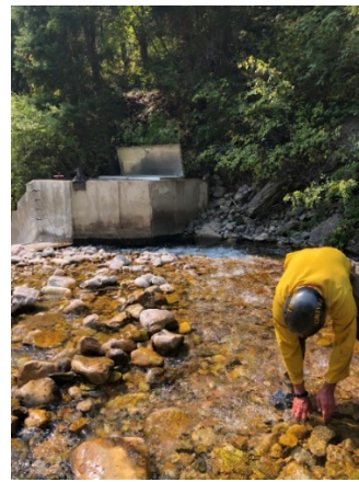
Rocks moved to direct more flows to diversion
