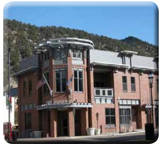
Figure 7-2: The new Fire Station 2 located in the Downtown
