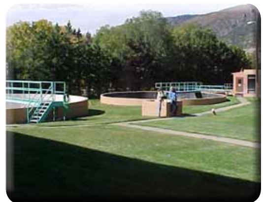
Figure 7-3: The site of the existing wastewater treatment plant near the confluence of the Roaring Fork and Colorado rivers
