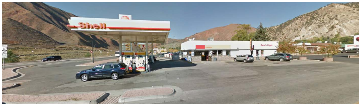
East elevation (Google Maps)
