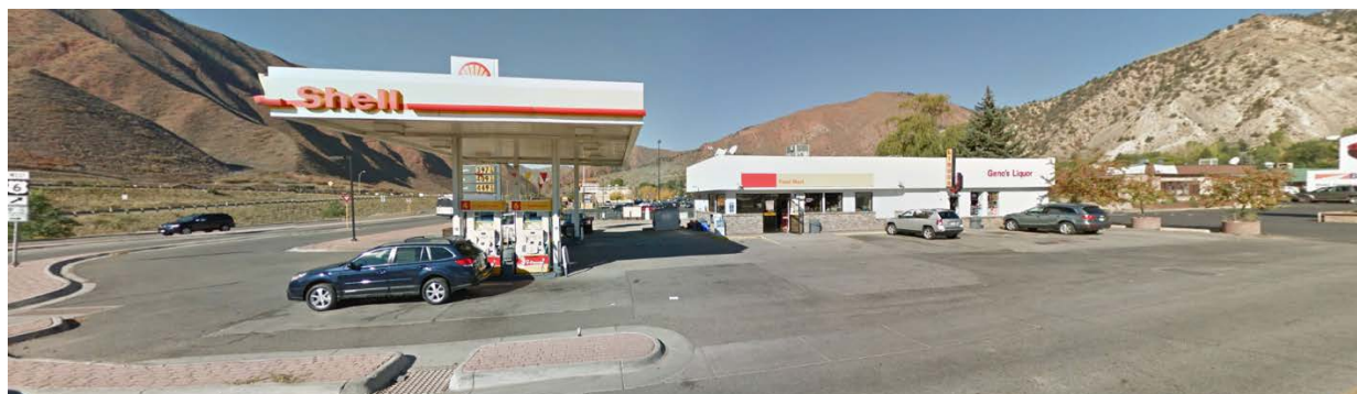
East elevation (Google Maps)
