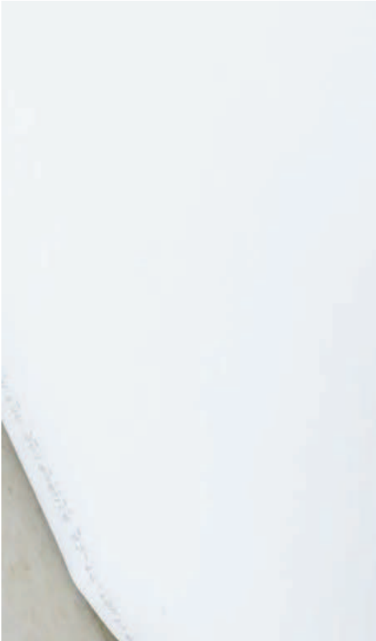
EPO ROOF OVER CONCRETE: WHITE
