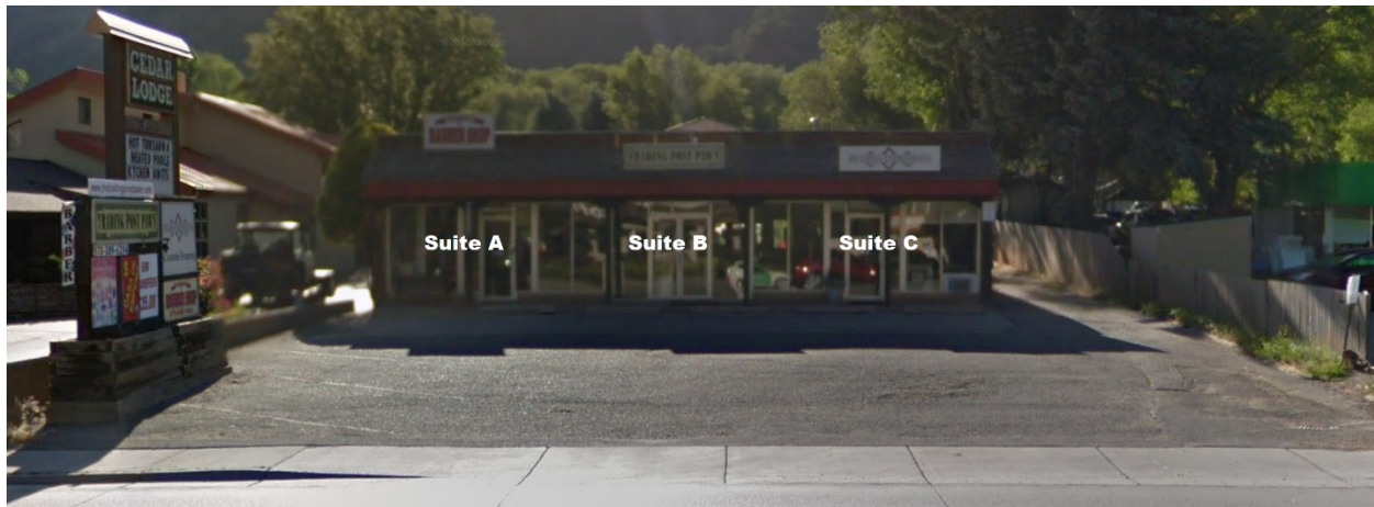
Figure 2. Front Façade Units
