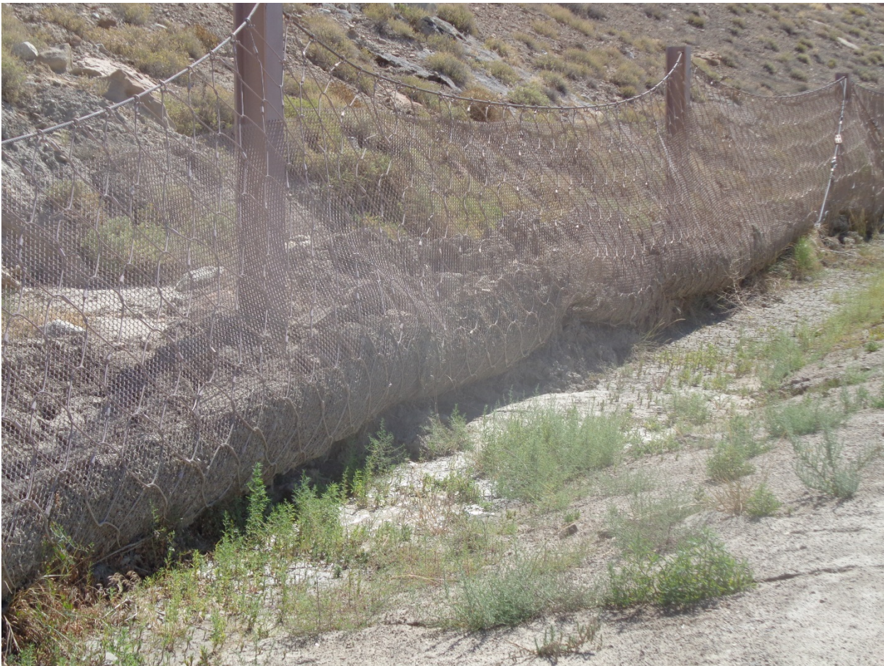
Figure 1 Flexible Debris Flow Fence Example
