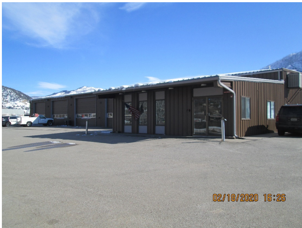
2222 Devereux Road showing existing building.
