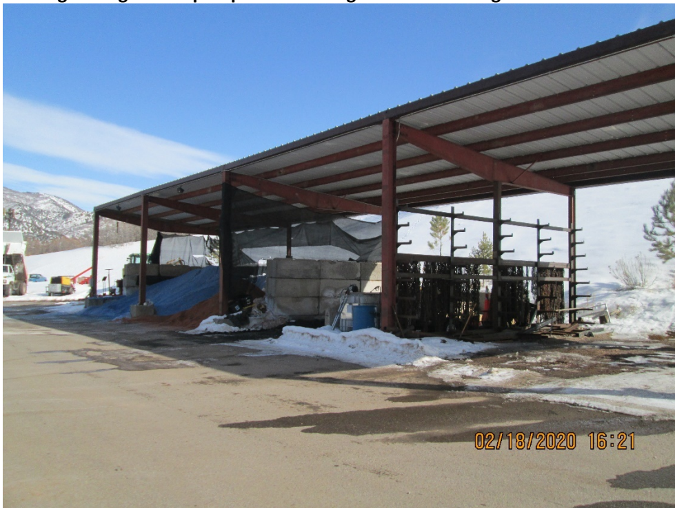
Existing MOC covered storage.
