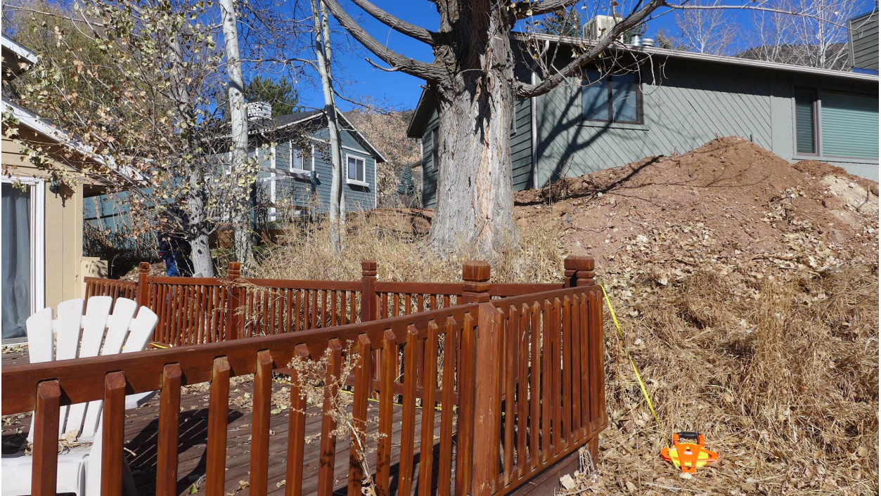
Looking north to Pittman residence from 546 Traver Trail. Excavated dirt reflected permitted work on Pittman deck.
