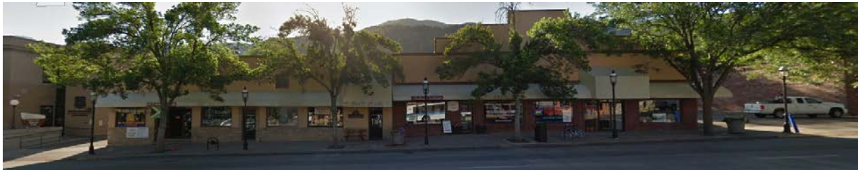
Existing west elevation (photo credit: Google Maps)
