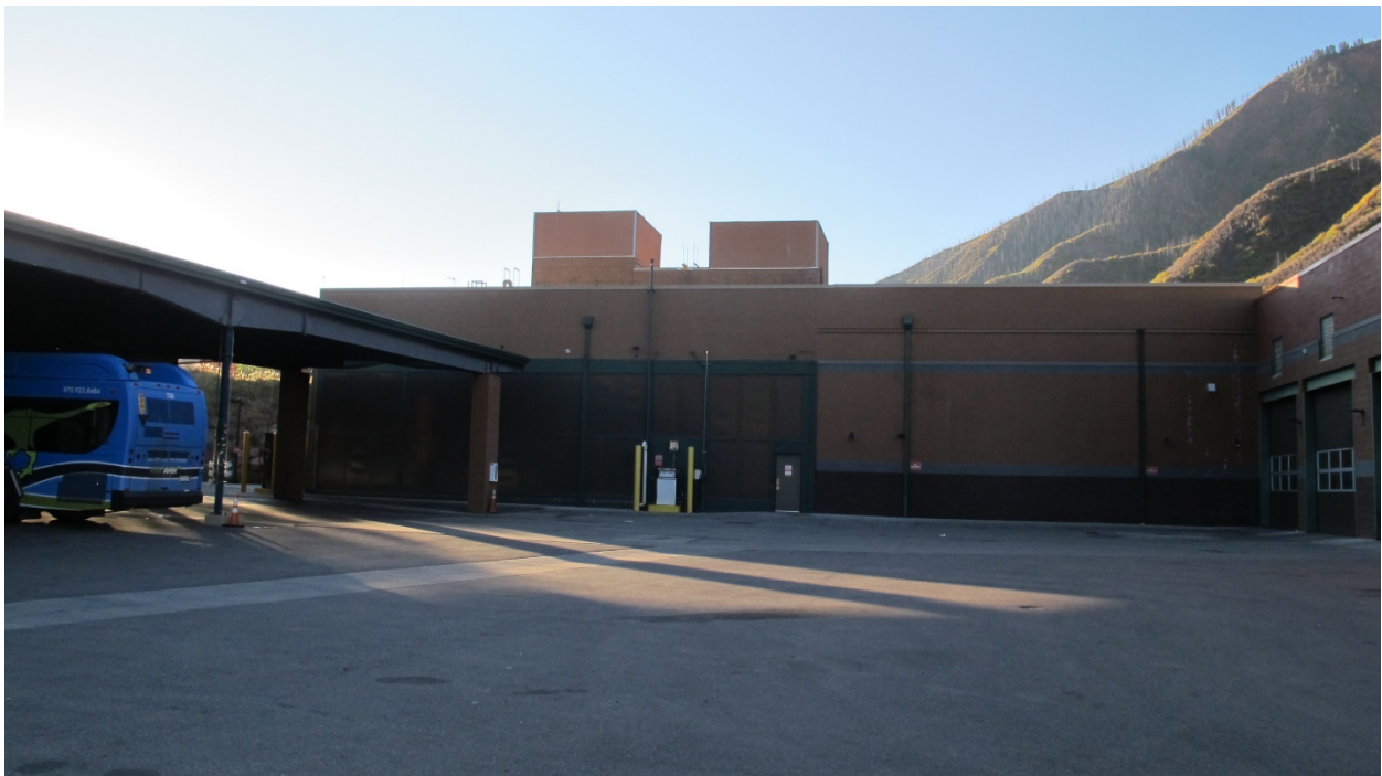
Photo 8-Canopy, looking from the north.
