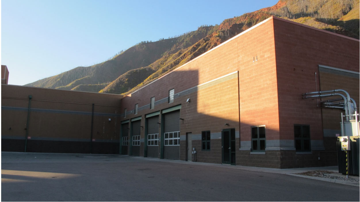
Photo 5-Maintenance bay exists, looking to the southwest
