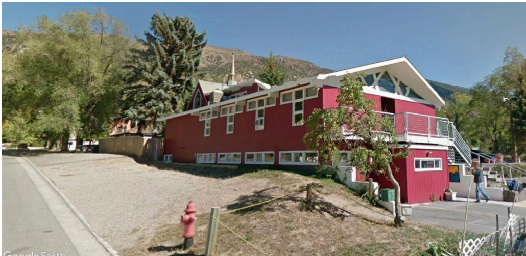
Source: Google Earth. Existing building showing south and west elevations.
